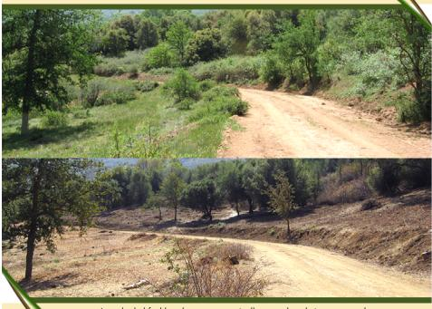
In a shaded fuel break, trees are typically spaced so their crowns no longer touch, lower branches are pruned, and brush and dead and down material are removed or replaced with masticated material. Shaded fuel breaks are most often placed strategically on ridgetops, roads, and around structures.
